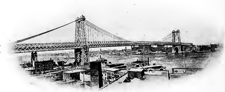
FIG. 43.—New East River Bridge.
